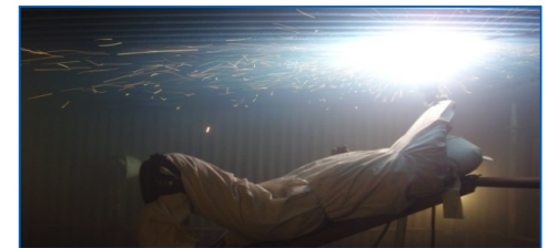
Application on boiler roof
